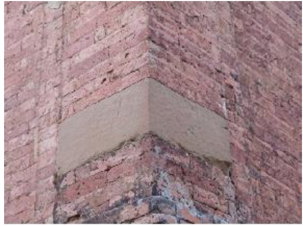
Reinforcement Sand Stone (Dhammayangyi Temple)
