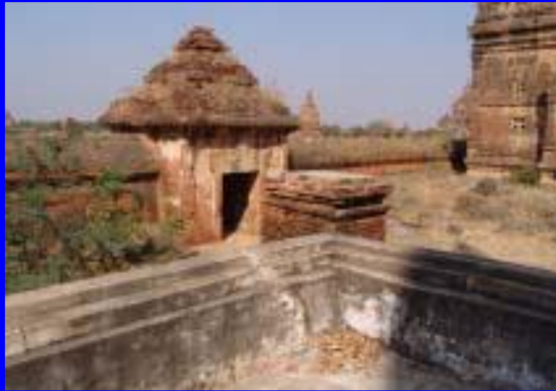
Double Enclosure Wall of Minnanthu Laymyethna Temple
