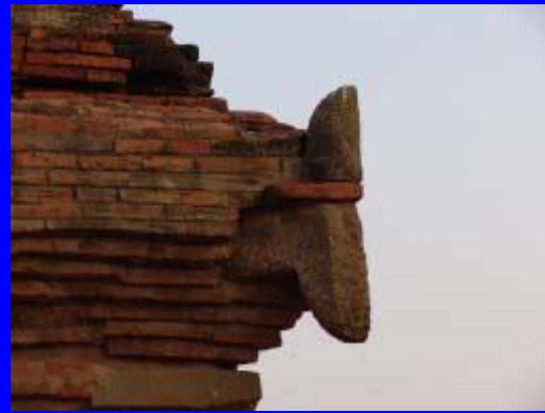
Reinforcement Sand Stone Mingalarzedi
