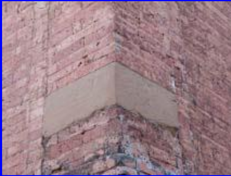
Reinforcement Sand Stone Dhammayangyi Temple
